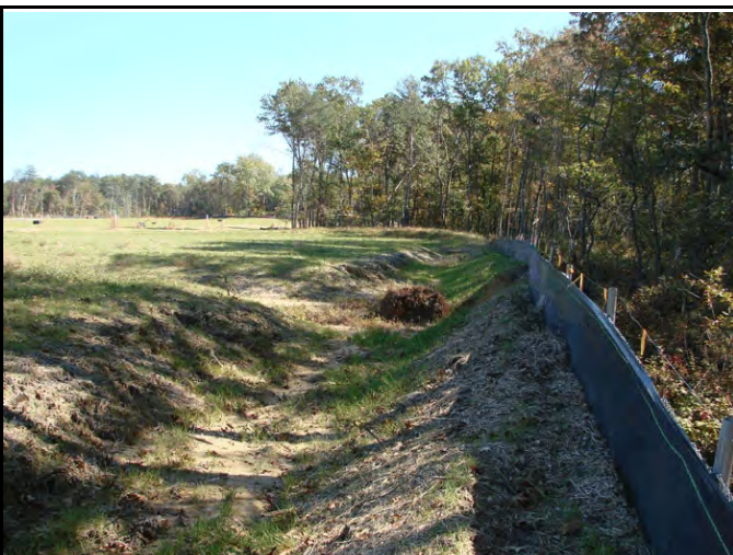
Perimeter Swale With Silt Fence on Dike Top
