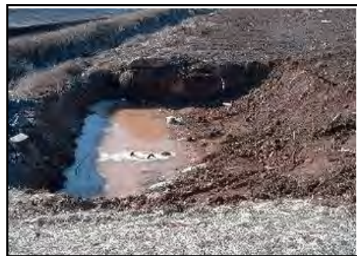
Sediment traps capture sand, some silt but little clay
