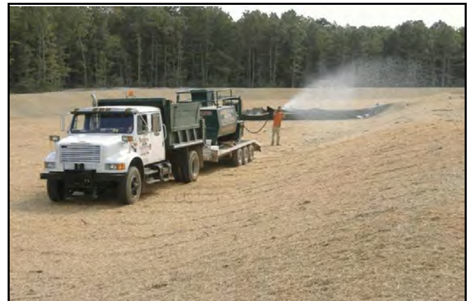
Hydroseeding: Applies Mulch, Grass Seed, Fertilizer & Water; Dense Growth in 4-6 Weeks
